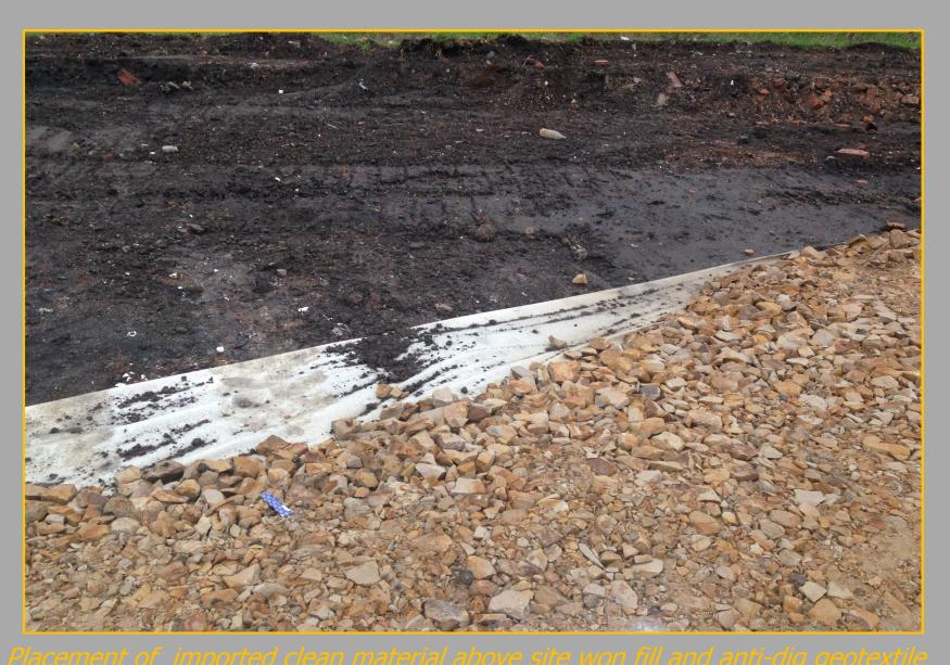
Verification consisted of nine trial pits in areas of soft landscaping to test samples of the topsoil and underlying imported material, to verify its suitability as clean cover material in-situ and verify that sufficient thickness of clean cover material is present across the site. Chemical testing confirmed suitability and each trial pit was excavated to a minimum of 0.65mbgl demonstrating that the thickness of clean cover exceeded the minimum thickness agreed with the LPA.
